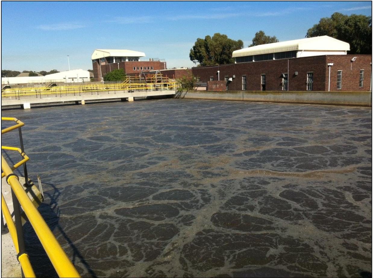
Figure 4: Fine-bubble aeration technology in an aerobic biological reactor at Athlone WWTP (July 2012) [Photo: M Grüter]
